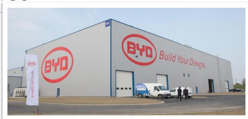
Bus assembly plant, Hungary: opened 2017
